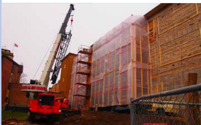
(Top to bottom) Workers remove the old cladding and replace it with new brick.
