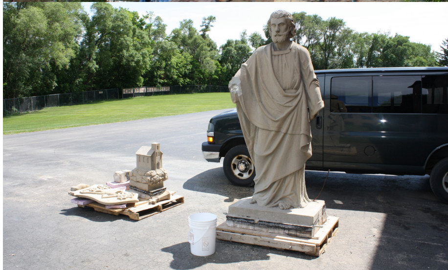
The statue of St. Joseph is being restored and will soon be replaced on the reconstructed portico.
